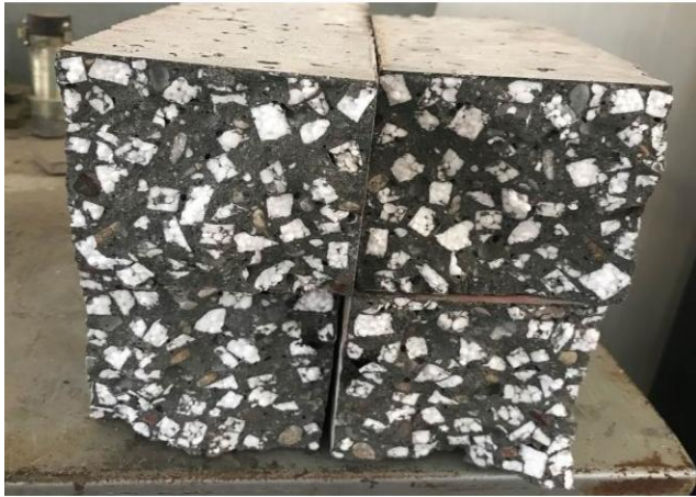
-b- sample failure
