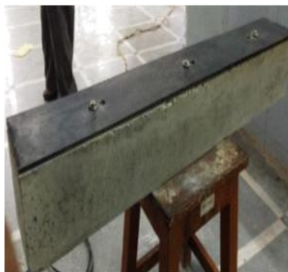
RCC Beam retrofitted with MS plates
